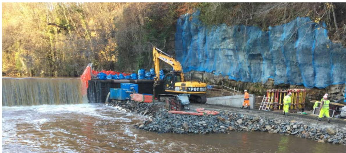
Meanwhile they have been getting on with the main works. Repairs have been completed to the weir crest, with replacement masonry filling the gaps that had appeared over the years. The additional water flowing through gaps of that type indicate a lower barrier height and attract the fish to try a jump. I saw a sizable salmon attempting just this a couple of months ago! It reached two-thirds of the way up but was not seen again.
