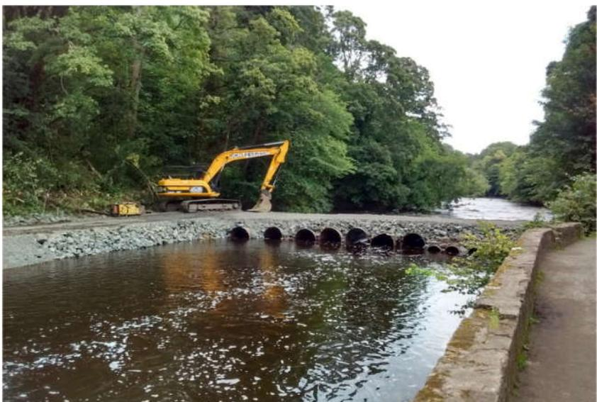
The Fair-a-Far weir has had a fish ladder since the 1970s, but it is in a sad state of repair and is no longer fit for purpose (or fit for fish). So work began in August this year to replace it with a state-of-the art 'larinier' fish pass.
